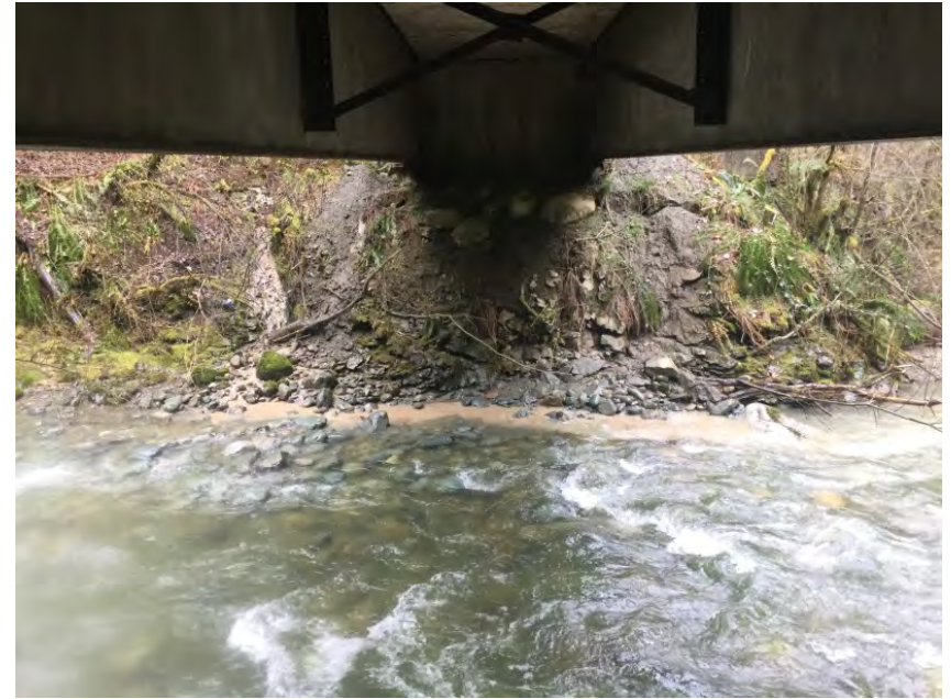
Left Bank Abutment when facing downstream
