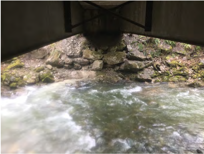
Right Bank Abutment when facing downstream
