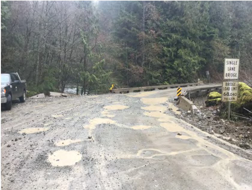
Approach from Right Bank when facing downstream
